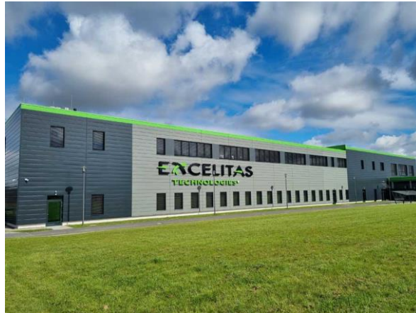
Caption image 3: The new plant offers extensive capacities for the assembly of optomechanical products in cleanrooms and clean zones
